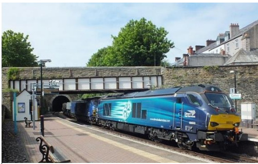
Figure 15 Limited structure clearance © Garry Stroud
